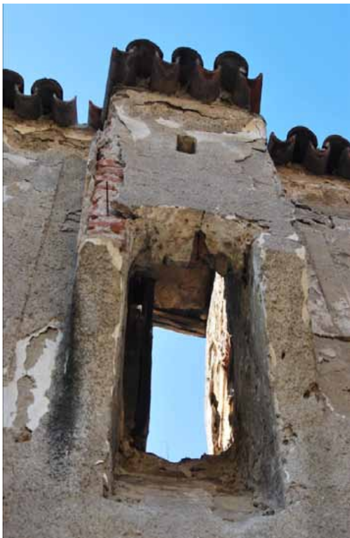
Dilapidated window in the fortified church in Cinso/Kleinscheck. Photo: Wikipedia
